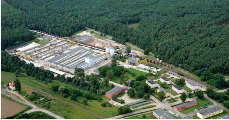
Prestressed Concrete Sleepers Manufacture
