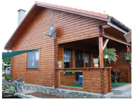
ZODAN – Wood Processing Plant (an example, one-storey house with a roofed terrace)
